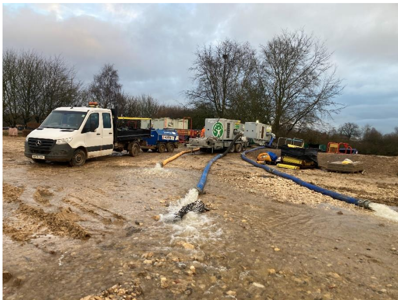
Photo: Temporary pumps taking water from Blue Beck
