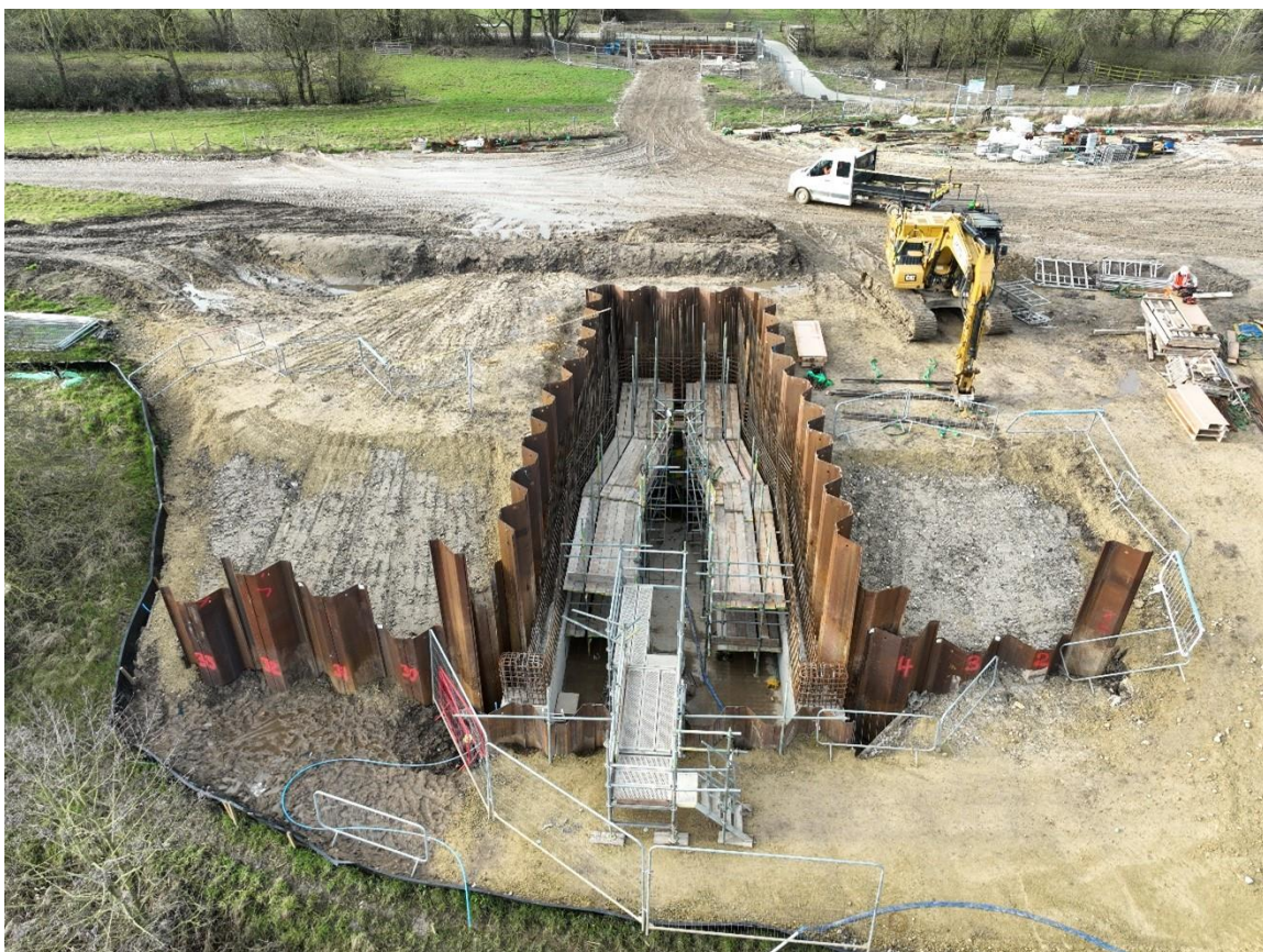
Photo: Building the structure for Blue Beck pumping station
